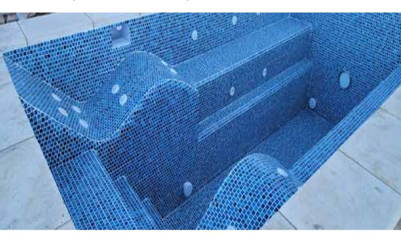
A power cord will need to be run into the footwell. Or, the cord of the LED Light will need to be extended. There should be a cavity to house 1m/3'6 of cord. This allows for the light to be serviced without the need of draining the Hot Tub. See separate section on LED Pool Light in this document. This refers to the LED light supplied by www.buildahottub.com – more information can be found at www.buildahottub.com/light
